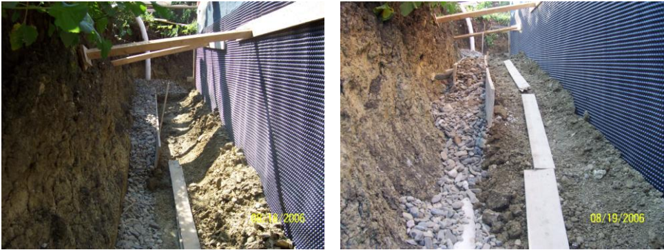
Fig. 4 – Placing the filter material on the drainage tube
