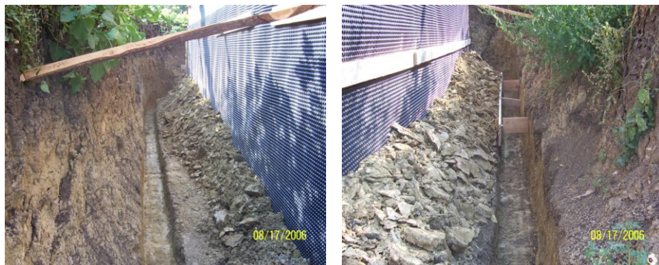
Fig. 2 – Channel execution for laying the drain
