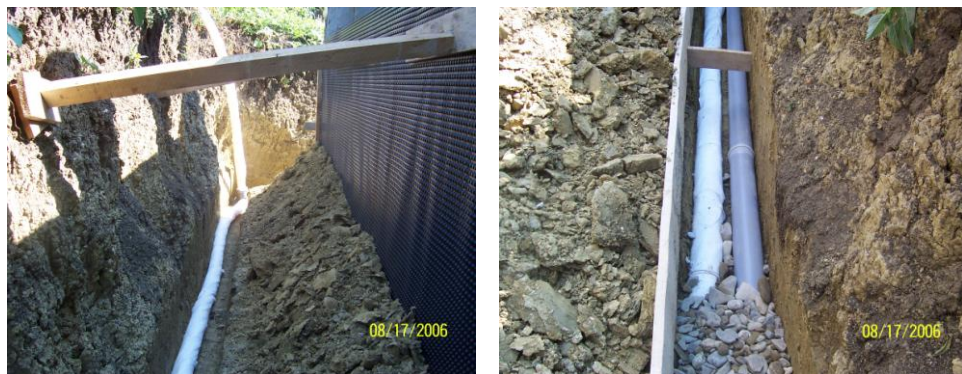
Fig. 3 – Laying the drainage tube wrapped with geotextile
